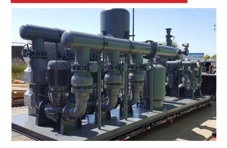
FlowTherm Systems™ pumping packages are designed for seamless installation. Whether for chilled water, hot water or condenser water systems, every package is pre-fabricated with all piping connections installed at optimum locations for smoothest operation. Control panels are available with VFD's and controller with single point power connections.
